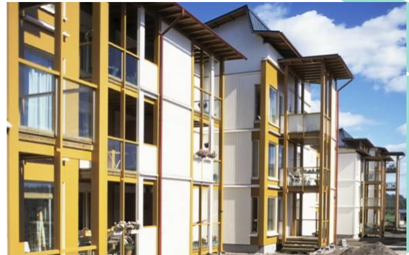
Viikki building Helsinki, Finland 21-flat building 1175 m 2 floor area
